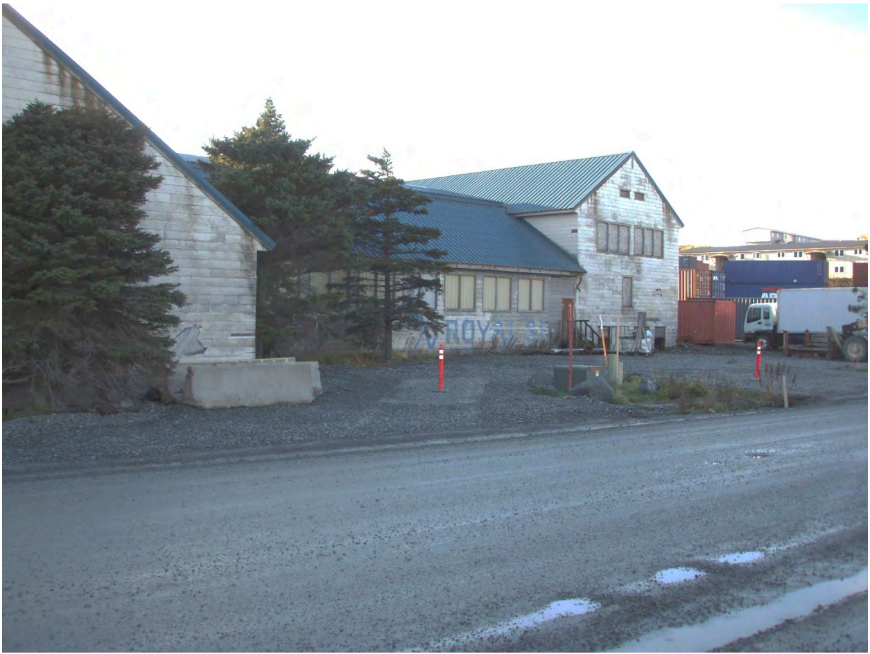
Photo 8: Front of Building 551 showing utilities and roadway. View looking northwest.
