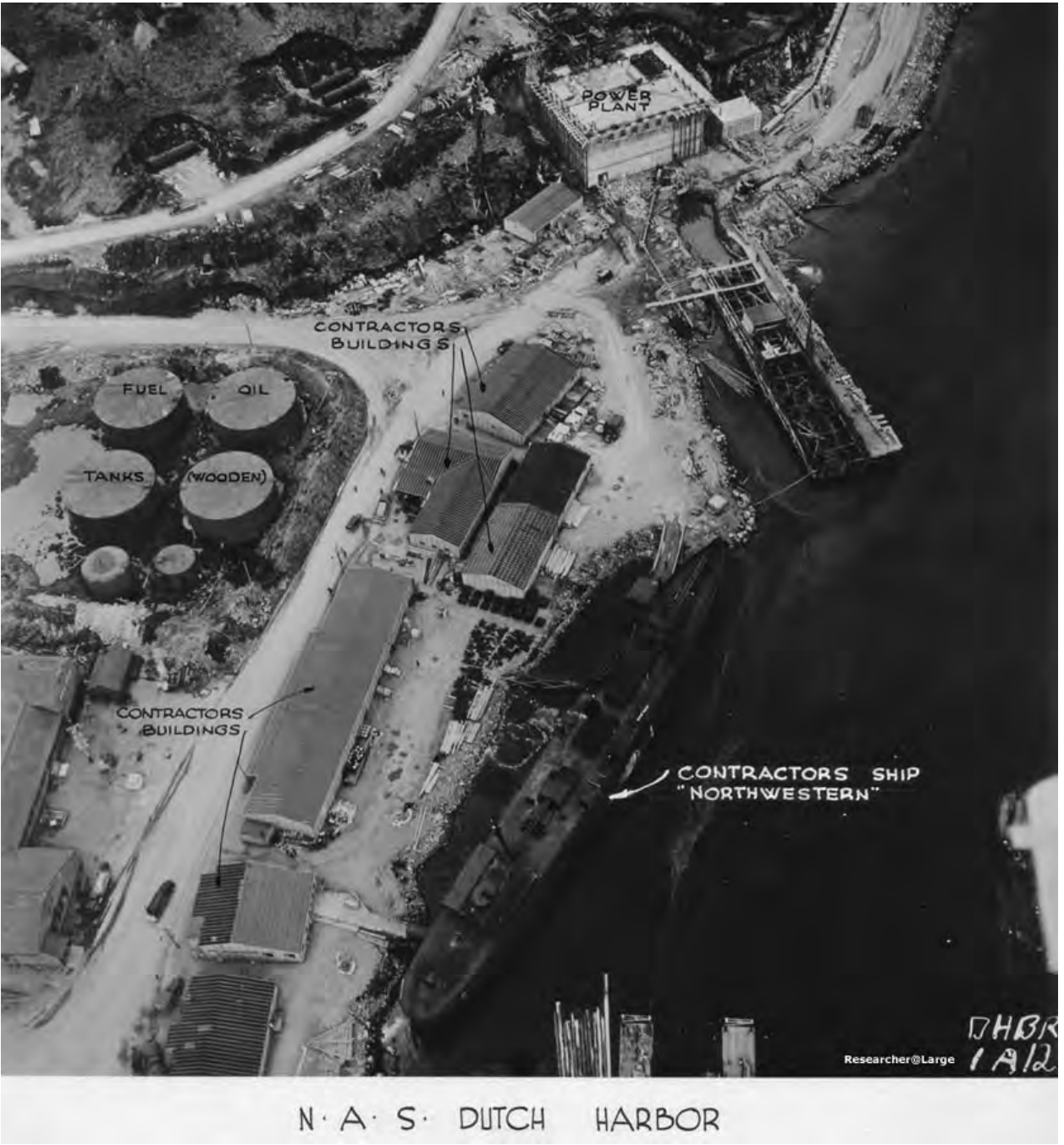
Photo 2: Historic photo prior to bombing. Navy Mess Hall at left Northwestern is tied along shore. Wood stave oil tanks and three transformers on poles are visible. View looking north.
