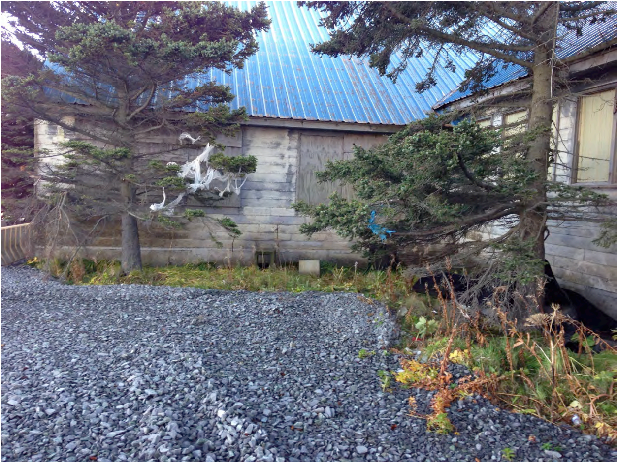
Photo 11: Front of Building 551 looking southwest.
