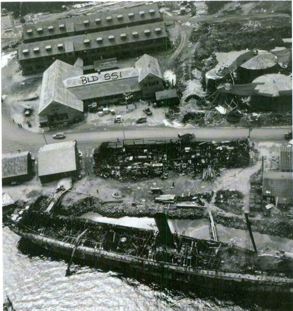
Photo 5: Historic photo after bombing. MV Northwestern is damaged and supply building destroyed across from Building 551. Three transformers still on poles in front of Building 551 may have been damaged. View looking west.
