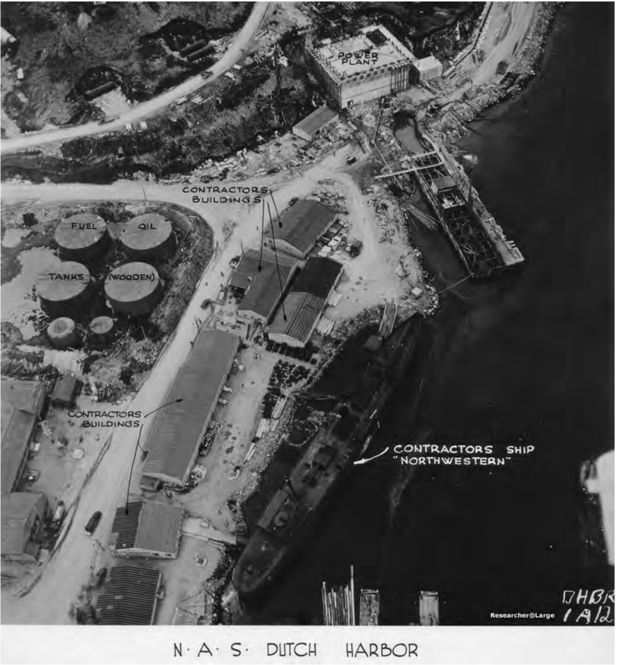
Photo 2: Historic photo prior to bombing. Navy Mess Hall at left and MV Northwestern is tied along shore. Wood stave oil tanks and three transformers on poles are visible. View looking north.
