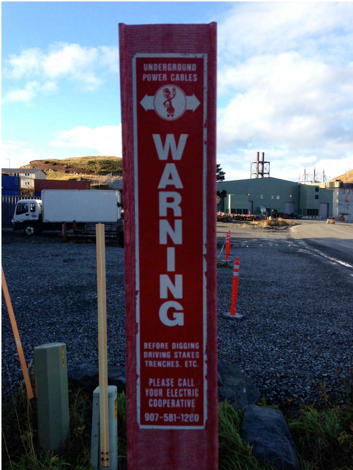
Photo 13: Call before digging signage: power
