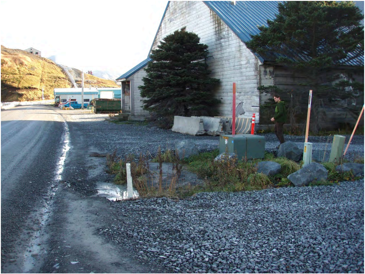
Photo 9: Front of Building 551 featuring utilities, roadway and entrance. View looking southwest.
