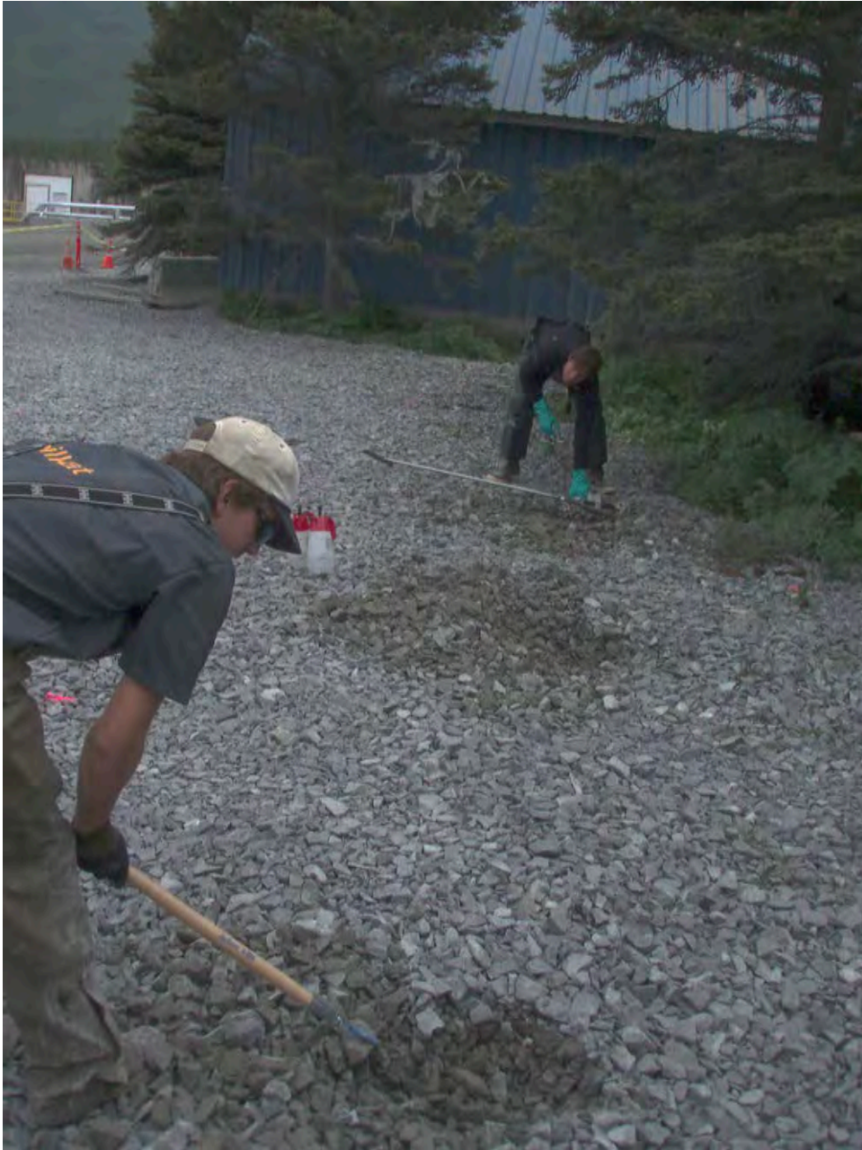
Photo 1: Clearing shot rock at sample locations
