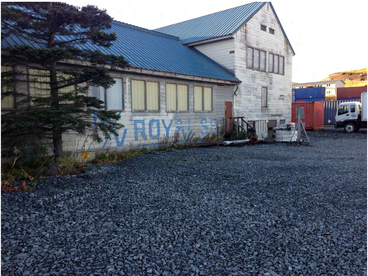
Photo 7: Front of Building 551 featuring recent gravel cover. View looking northwest.
